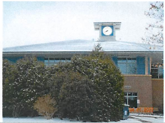
4. Partial view of the north roof. Reference Photo #6 for IR image.
