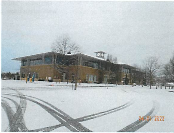
1. Overview of the south and east elevations of the facility.
