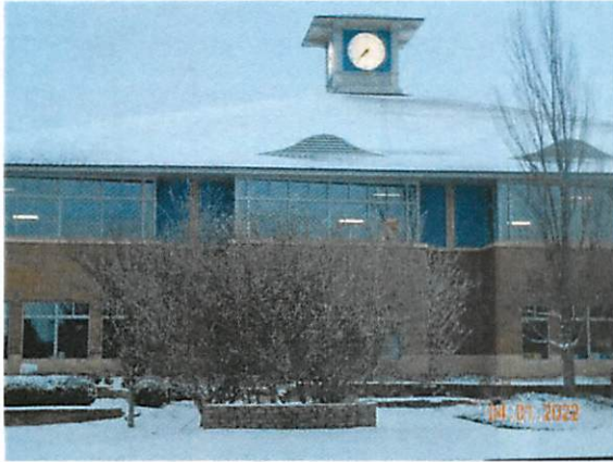
7. Partial view of the west roof. Reference Photo #9 for IR image.
