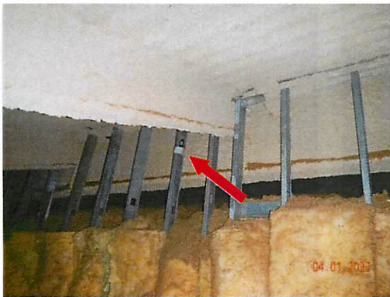
21. View of Data Logger #3 placed towards the upper portion of the unconditioned side of the south 3 rd floor mezzanine wall.
