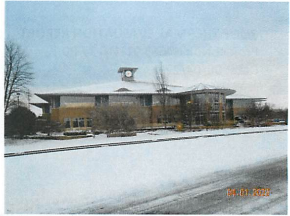
2. Overview of the west elevation of the facility.
