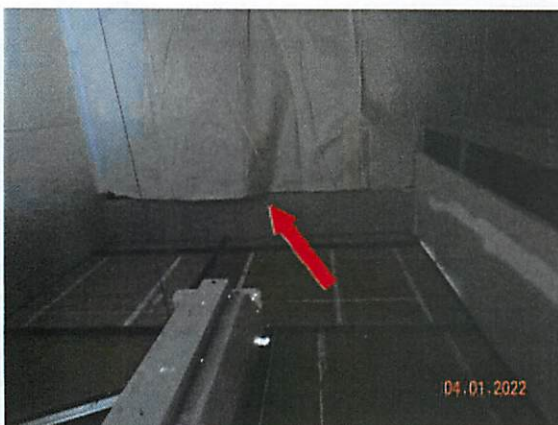
41. View of open interface lap of the plenum air/vapor barrier in the south plenum.
