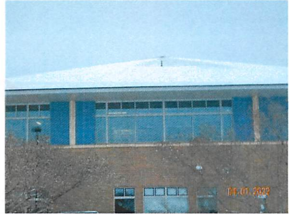
8. Partial view of the south roof. Reference Photo #10 for IR image.
